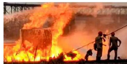
Firefighters try to control the blaze that broke out in a Haldia Petrochemicals pipeline in West Bengal on Tuesday. PTI
